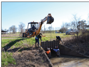
Crew Installing Box Culvert Weir in Valewood Ditch
